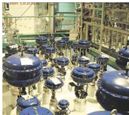
Velan Adareg Cryogenic Control Valves for Liquid Helium at 1.8°C above absolute zero, specially designed for the world's largest particle accelerator at CERN, Geneva.
