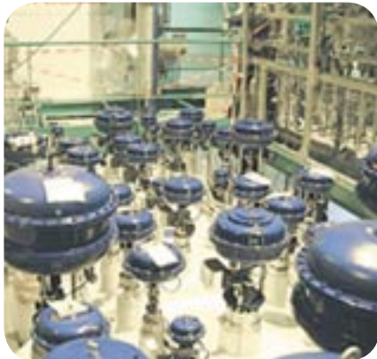
A custom-made Velan product for the world’s largest particle accelerator in Geneva: low-temperature valves for liquid helium at 1.8°C above absolute zero.
